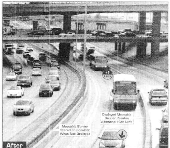
Deployed barrier creates additional lane in the peak direction - Dallas, Texas, USA
