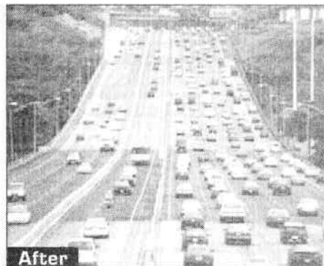
QMB-RTS borrows lanes from underutilized side and adds lanes to peak traffic side - Honolulu, Hawaii
